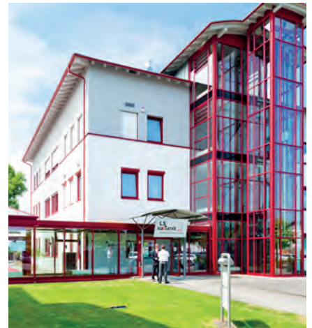
LS telcom Training Academy in Lichtenau/Germany
